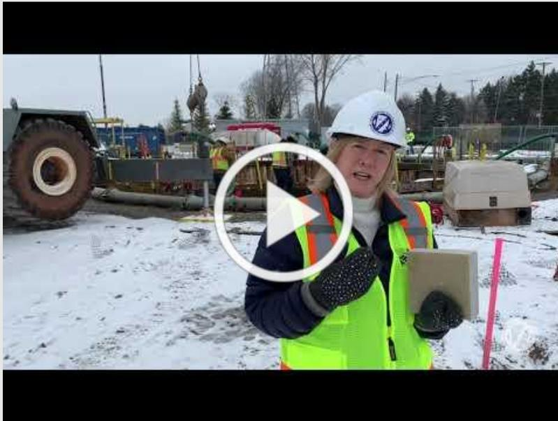
Remember the 2016 sinkhole event? Well, construction is now underway on a two-year, \$28 million project which will prevent future infrastructure disasters from occurring in that stretch of the Macomb Interceptor sanitary sewer. A construction firm is digging a 65-foot-deep shaft in the ITC Corridor, west of Schoenherr Road, to reach the massive sewer that carries the waste flushed by more than 500,000 people from nearly a dozen communities in Macomb County.
